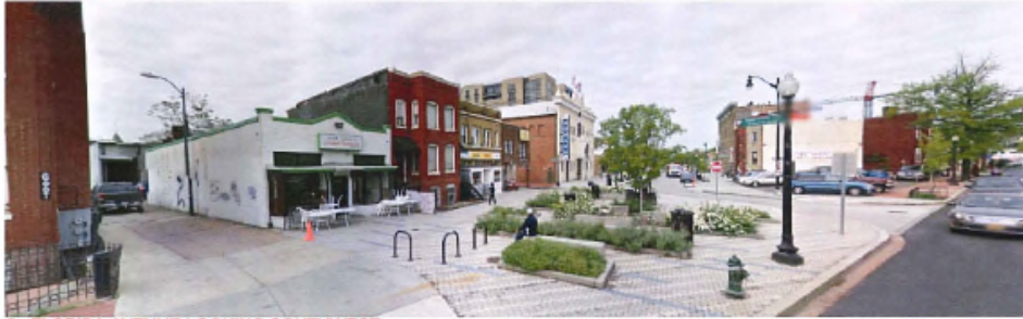
2 - FLORIDA AVENUE LOOKING SOUTHWEST
