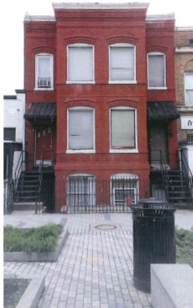
610 T ST, NW LOT 352 A PORTION OF THE BUILDING TO BE INCORPORATED INTO THE PROJECT
