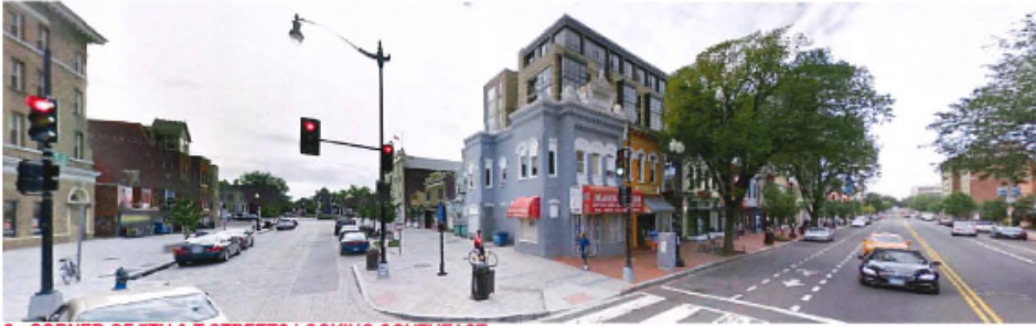
2 - CORNER OF 7TH & T STREETS LOOKING SOUTHEAST
