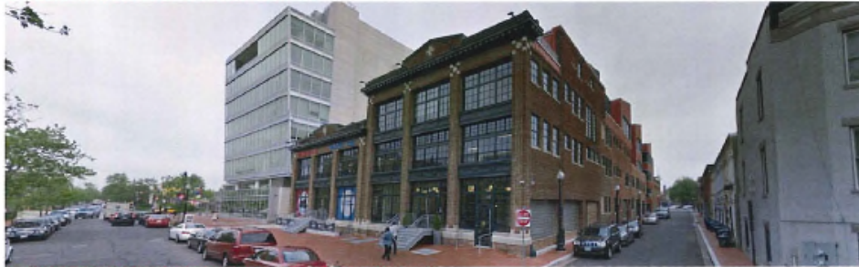
3 - S STREET LOOKING NORTH DOWN WILTBERGER STREET
